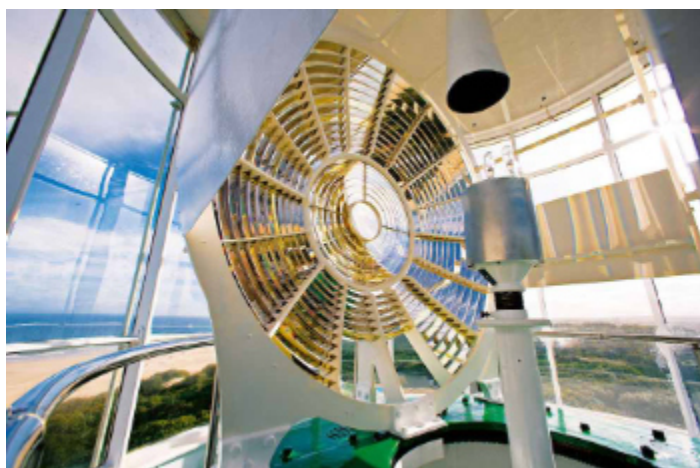
Inside the 1st Order, two-panel Chance Brothers dioptric rotating optic, with the 400-Watt metal halide lamp.
